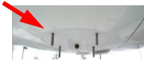
Figure 2.21: Mounting pad installation on radome base.
