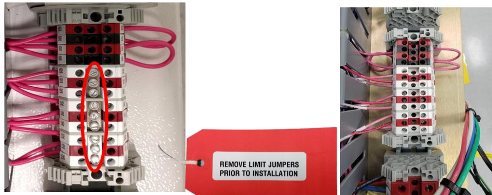
Figure 3-22 Remove limit jumpers to be removed ( left installed ) ( right removed )
