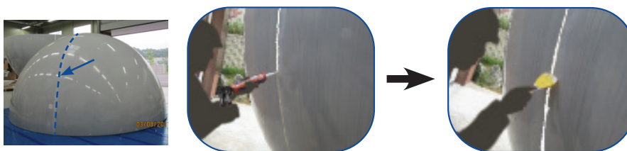
Figure 39: Spreading Silicone between Radome Panels
