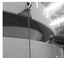
Spread Silicone on Surface
