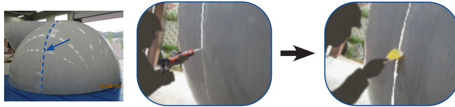
Figure 41: Spreading Silicone between Radome Panels
